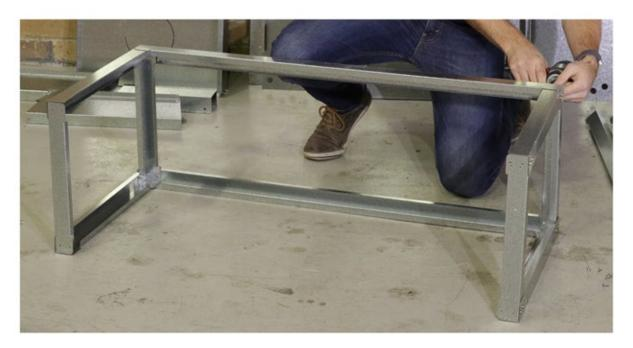
Once you have completed the top two rails, turn the frame over and repeat the process for the lower long rails to complete the base.
